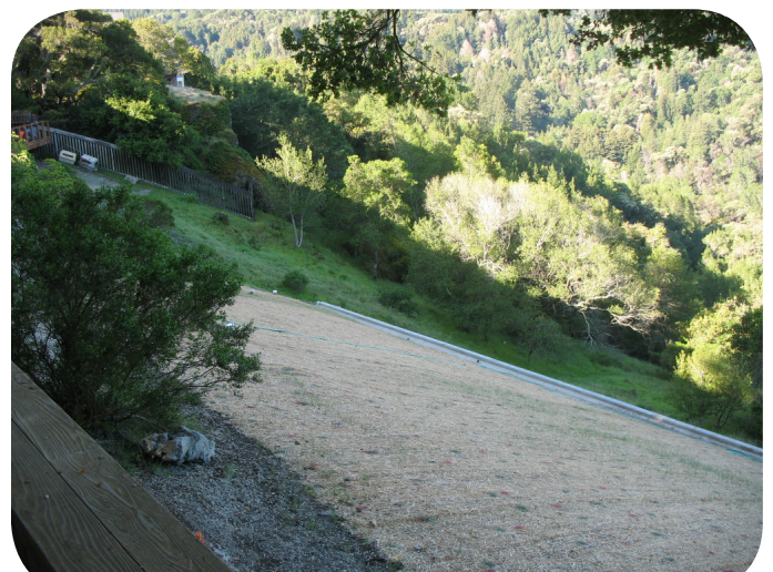
Finished slide repair. Hillside re-seeded and erosion protection matting installed.
