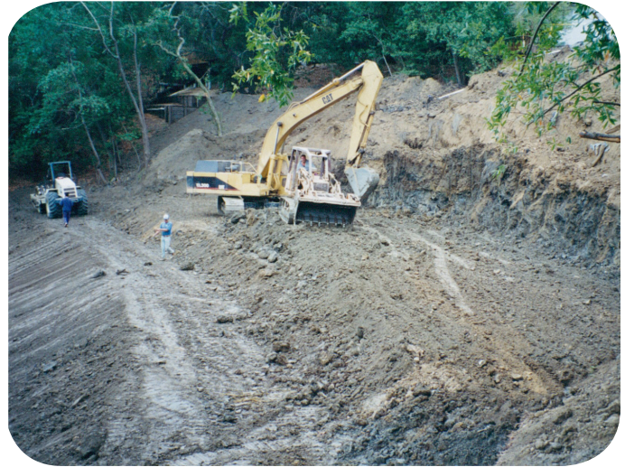
Spreading out slide material in 8" lifts
