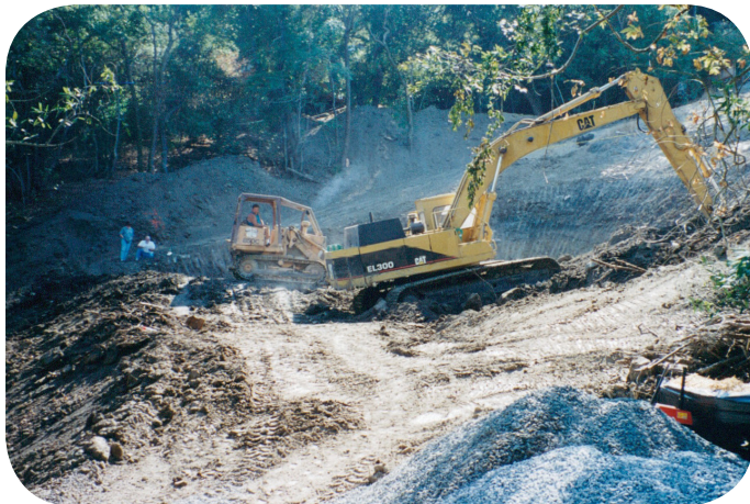
Excavating out unstable soils
