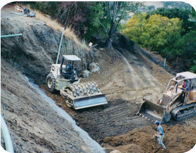
Compacting slide material with sheep-foot roller. Top of sub-drain gravel showing.
