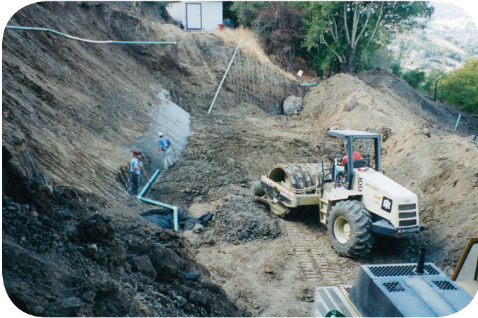
Drain pipe and sub-drain installation, with sheep-foot compactor in foreground
