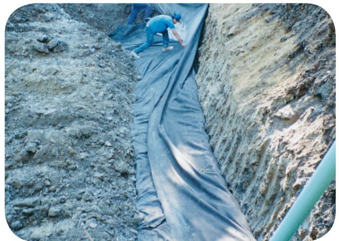
Wrapping a sub-drain at the back of a bench, in filter fabric
