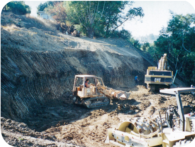
Working our way up the hill, excavating a bench into competent material
